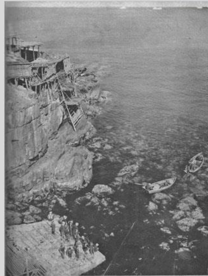
From Open Boat to Cleaning Shed, Cod Climb Pouch Cove Cliffs, Platform by Platform When the vessel is in, fishermen stand on cliffs above, like miners on open benches or ladders in a backfill, and pitched the heavy cod from step to step. Though the structure looks flimsy, its steel girders, main beam and cap run after rear. Rode down through the clear water. Business stand on the feet of their ramp (page 181).
